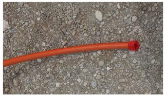
1.1 During installation of micro duct bundle a temporary sealing cap should be used. After laying micro duct bundle straight in the trench, temporary sealing cap can be removed.
