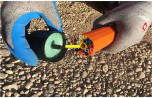
1.5 Position central thorn in front of central tube from micro duct bundle.
