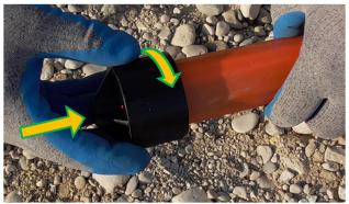
1.6 Press sealing cap on duct bundle and turn it clockwise all the way till stop (hand-tight).
